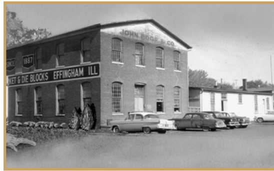
JOHN BOOS & CO. WOOD MANUFACTURING FACILITY EFFINGHAM, IL
