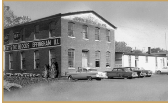
JOHN BOOS & CO. WOOD MANUFACTURING FACILITY EFFINGHAM, IL
